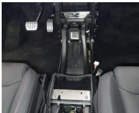
Figure 46. Center console HVAC duct
